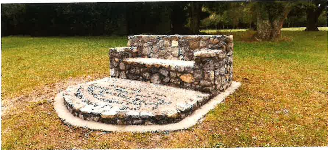
The completed Walkway gathering point and the quote from St Bernard is formed in the concrete with letters/words in stones. (above)
